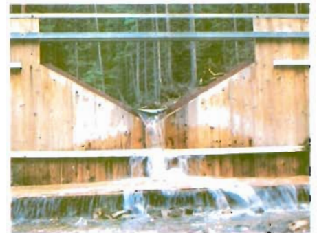
The height of water tumbling through this "V" shape acts as a gage of water runoff at the experiment station near Fraser.
